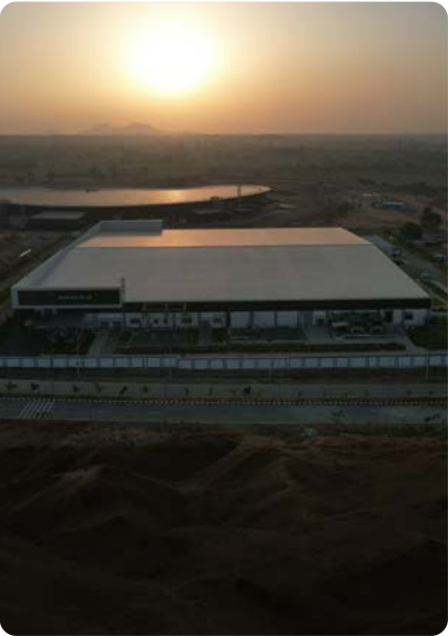
Under construction Giga Corridor
